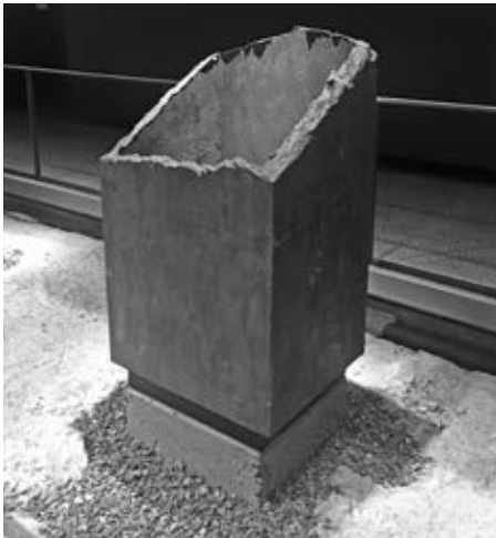
Box column remnants
