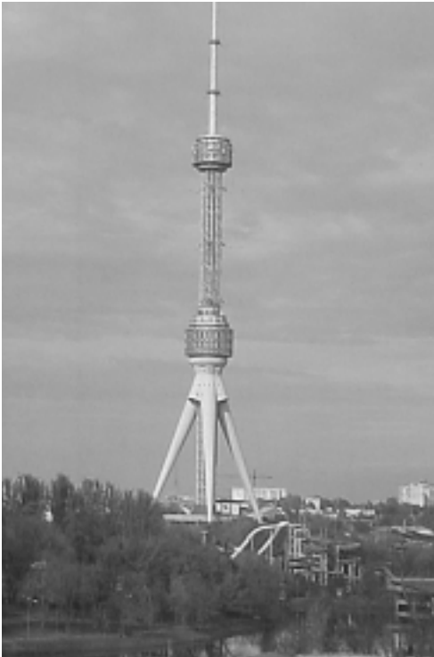
Landmark telecommunications tower in Tashkent
