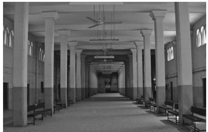
Mosul Court before rehabilitation
